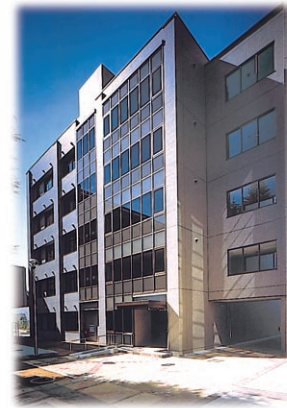
総合研究棟 H棟 H Hall (Integrated Projects Research Center)
